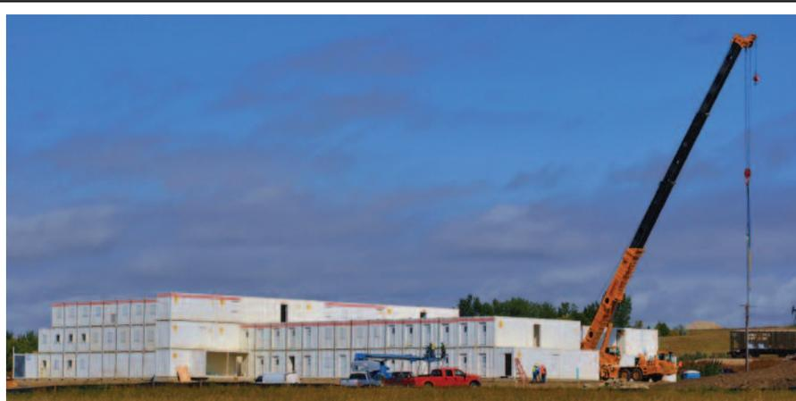
With a scarcity of housing and hotel space, one solution is temporary units designed to provide comfortable accommodations for oil field workers. Shown here is the Muddy River Lodge, a three-story, extreme weather complex constructed from rail containers that houses 300 Halliburton employees.
